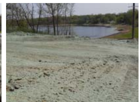
Temporary stabilization during construction to protect water resources
