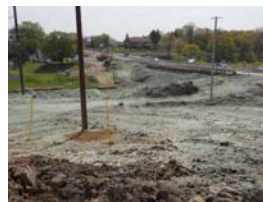
Temporary stabilization during construction to protect water resources
