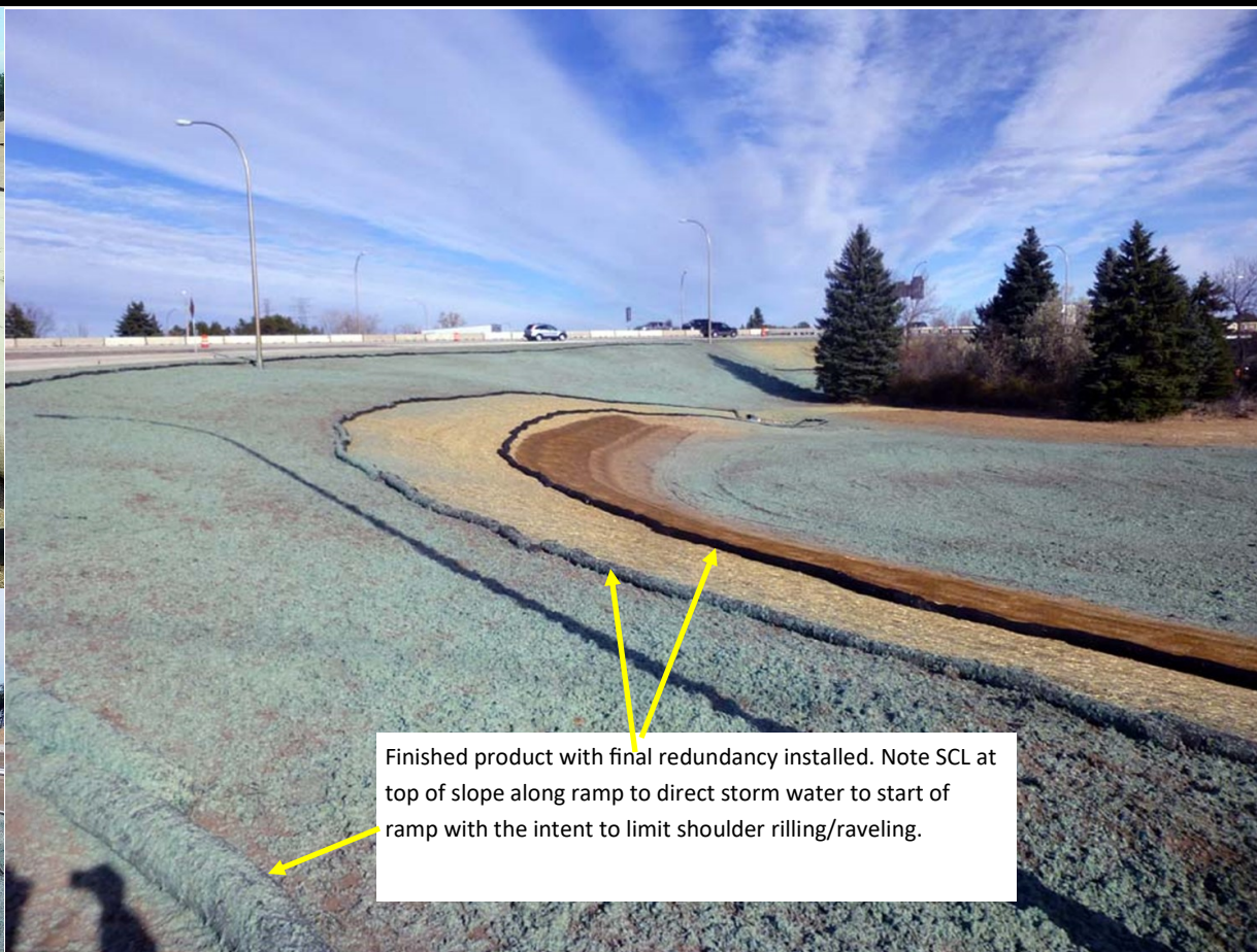
First prepare topsoil soil, fertilize, till, seed and stabilize prior to installing additional redundant perimeters
