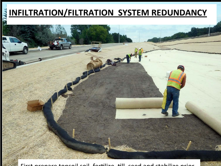
First prepare topsoil soil, fertilize, till, seed and stabilize prior to installing additional redundant perimeters
