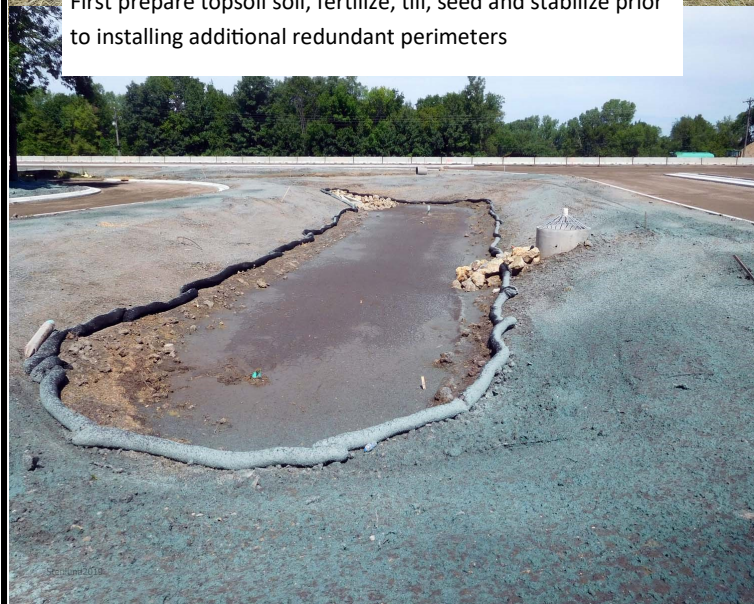
Critical first line of stabilization blanket basin ring and sediment control redundancy.
